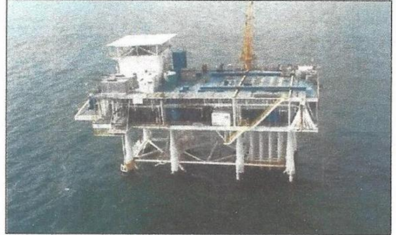
Photo before the mudslide toppled the platform in 2004.
