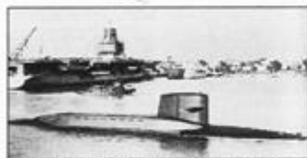
1960 photo of CVAN-65 under construction, with USS Robert E. Lee (SSBN-601) departing for sea trials
