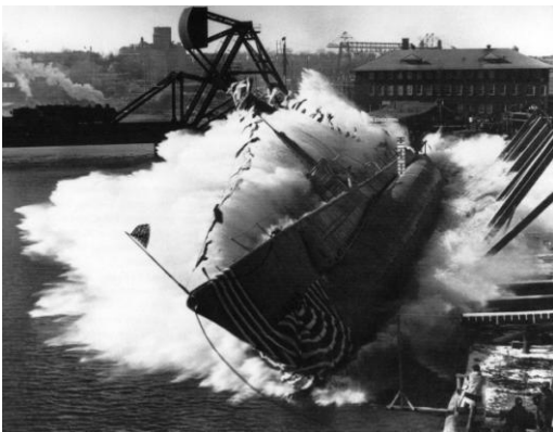
Figure 2 depicts a submarine being launched into the Manitowoc River by being tipped over sideways as can be seen with a huge splash of water. This method of launching had no problems with the builder.
