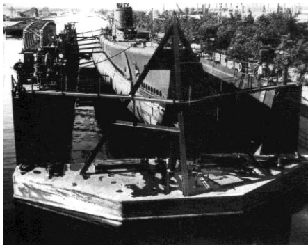
Figure 3 illustrates the special dry-dock loaded and ready to transport a submarine. This contraption was designed and constructed to carry the freshwater submarines from Lake Michigan to the sea.
